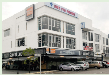
CHERAS SELATAN 118 @ BALAKONG 49 units, 2 Storey Shop Office + Mezzanine Floor, Completed in 2016
